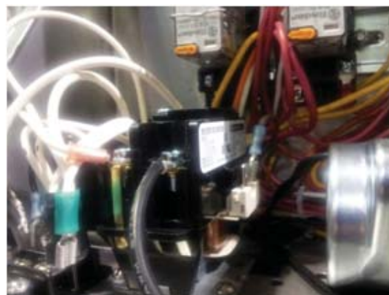
Wash motor contactor to the left of the cam timer motor
