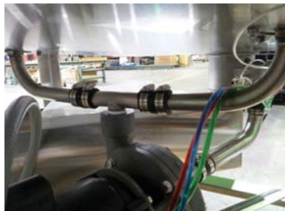
Pump discharge split/manifold
