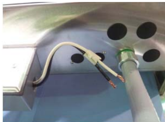
Showing power connection for 120v wiring
