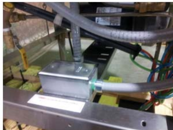
AFB connection box, the water inlet can be seen at left
