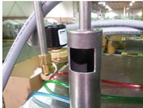
ASSE approved air gap (backflow preventer)
