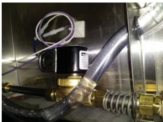
Showing \frac{1}{2} " H 2 O solenoid, also plastic drain tube
